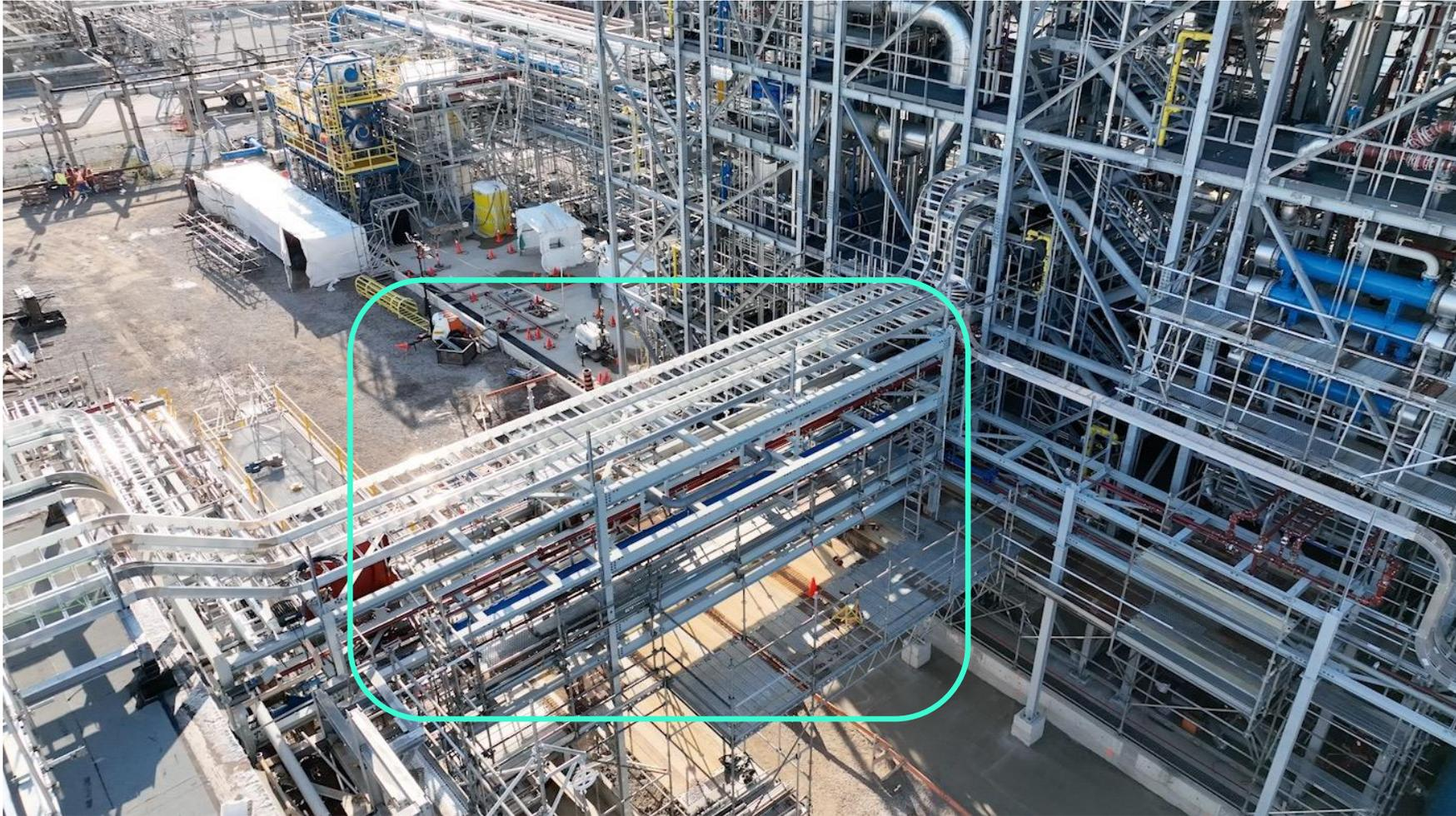
The main pipe rack connects the key production modules to the HTC building, tank farm, and power distribution building. This pipe rack delivers process chemicals to and from the tank farm and key production modules. In addition, it will supply electrical power from the power distribution building to the key production modules and ENCON evaporator module system.
