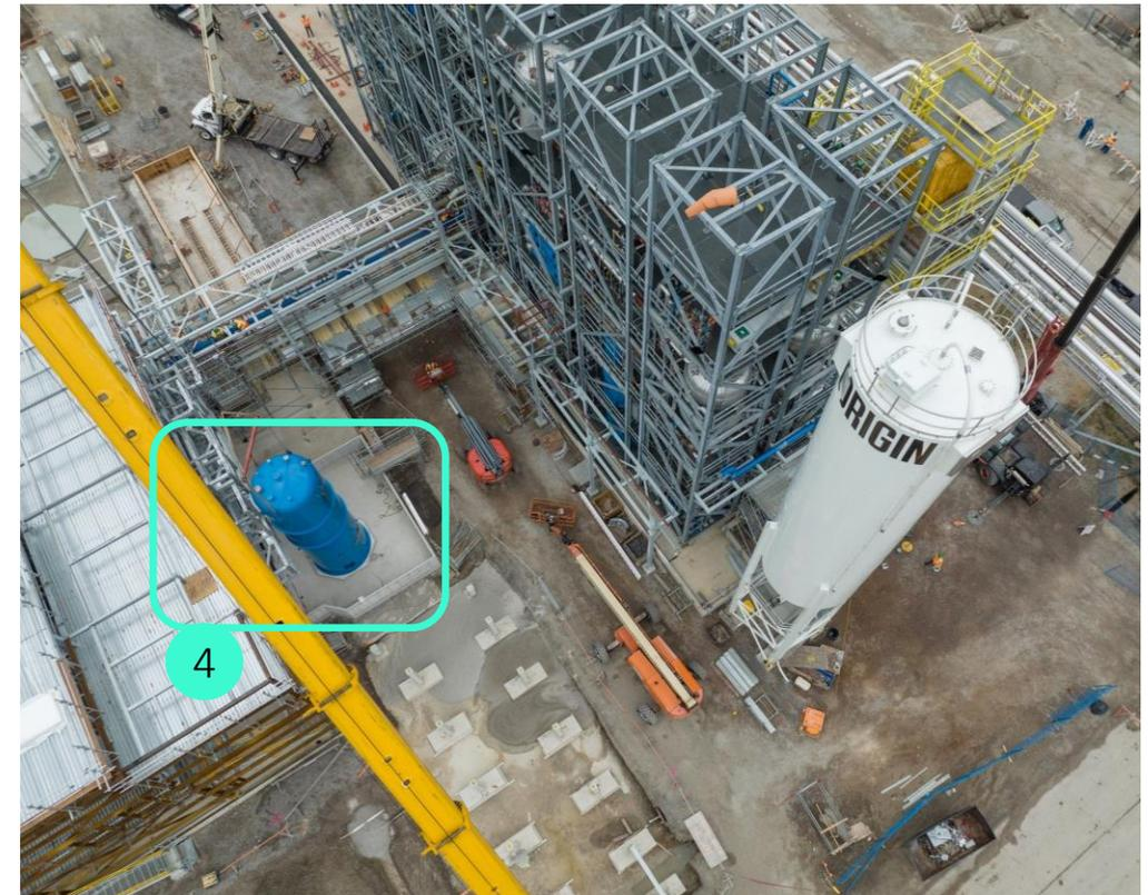
1. Storage tank for containing unrefined CMF before its distillation step. Due to its large size, our distillation feed tank was assembled onsite rather than delivered by road. The unpainted areas allow for welding. 2. Brine tanks and HCl tanks. 3. Solvent tanks and storage tanks for finished CMF. 4. Brine recovery tank
