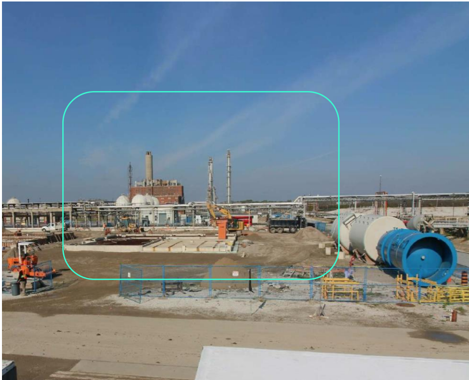
Pre Module Installation (Week of October 11 th , 2021)
