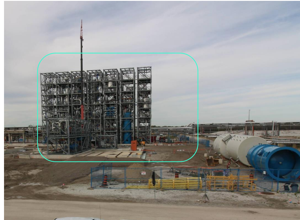
Post Module Installation October (Week of October 25 th , 2021)
