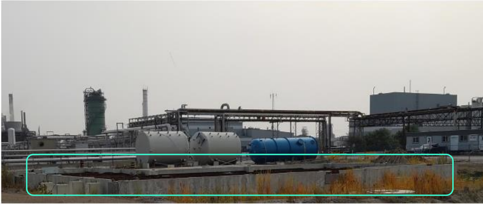
July 22 nd , 2021 (Foundation Perimeter Poured, Rebar Installed)
