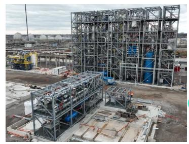
"After": Clockwise from top we see the biomass building, HTC building and filter press, solvent tanks, piping modules
