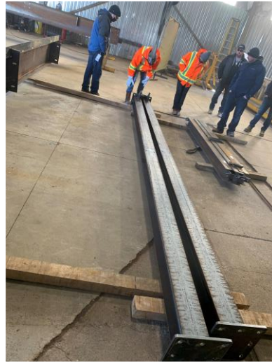
Finished steel verticals
