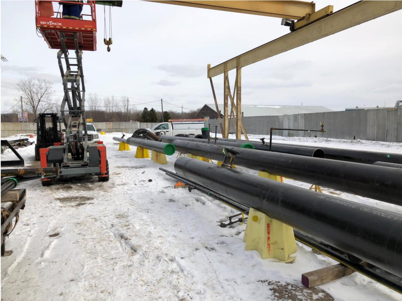
Pipe fabrication prior to painting
