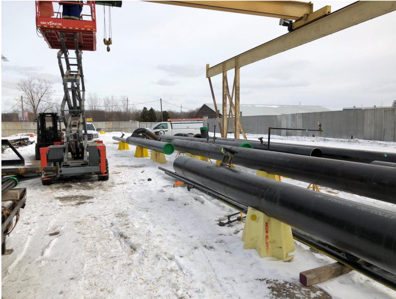
Pipe fabrication prior to painting
