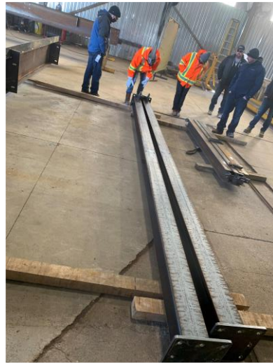
Finished steel verticals
