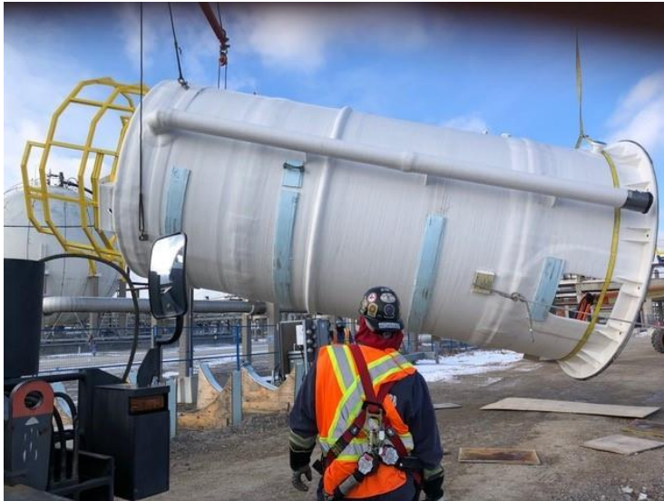
ENCON tanks being offloaded and placed
