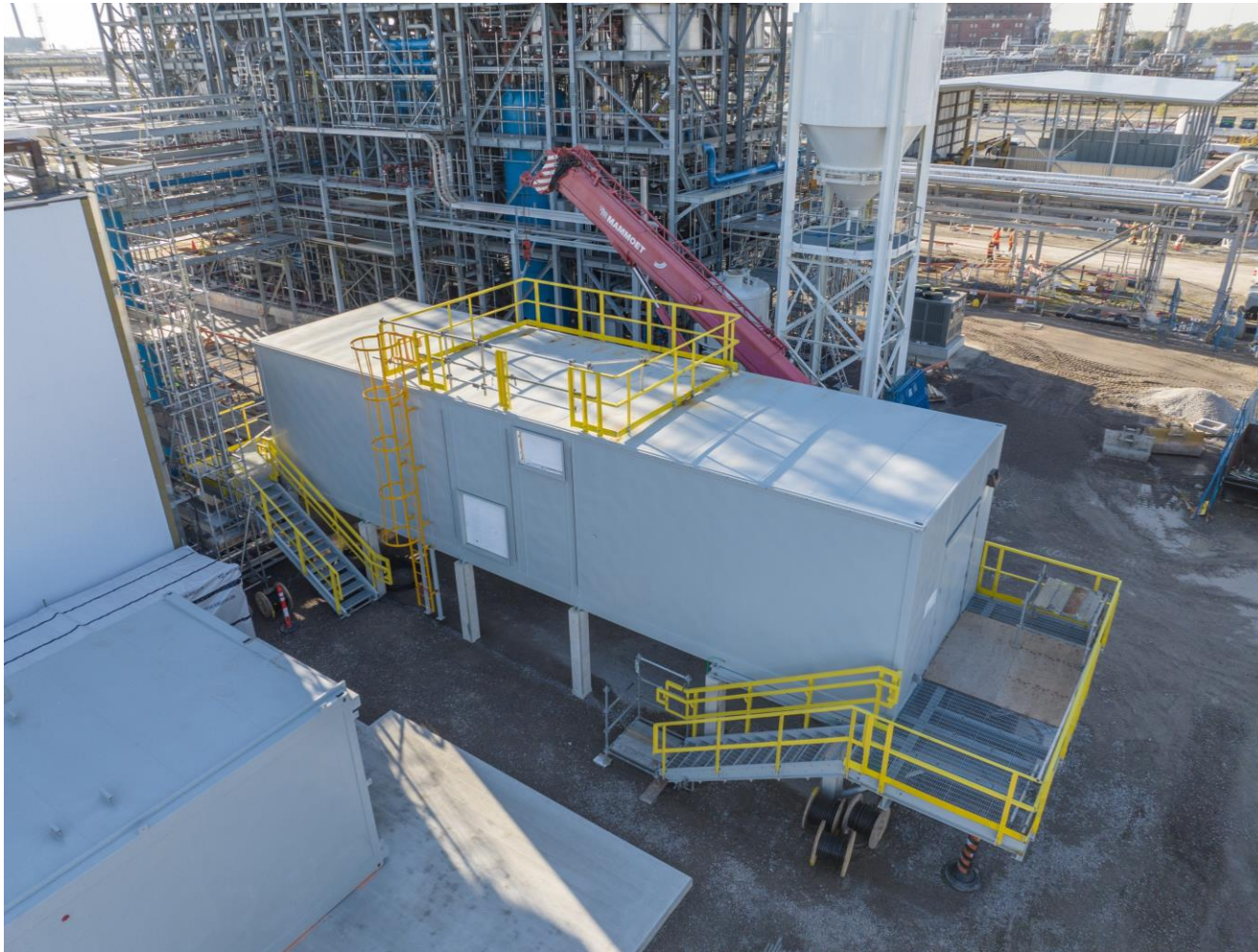
The power distribution building contains the motor control center
