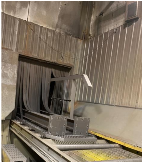
Blast cleaning steel verticals
