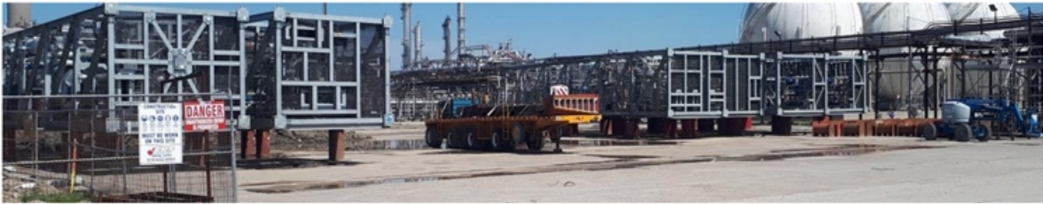
Core process modules awaiting installation
