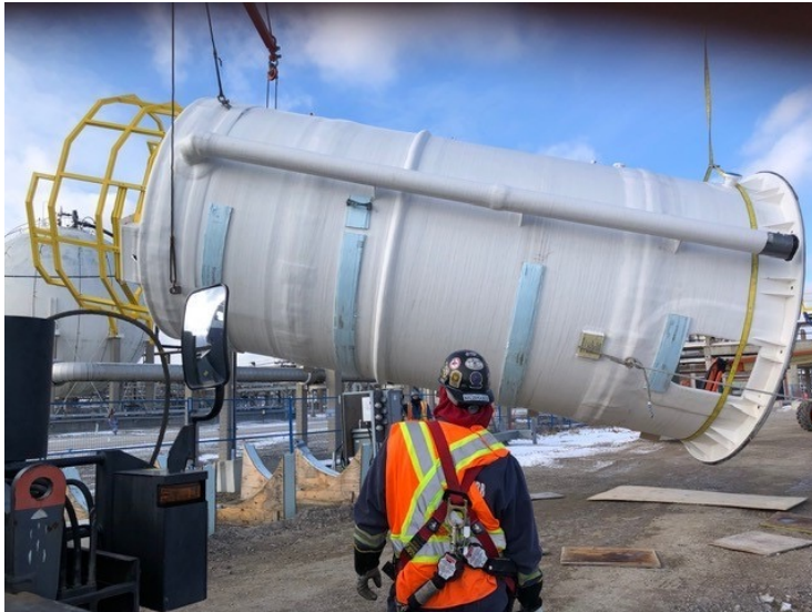
ENCON tanks being offloaded and placed
