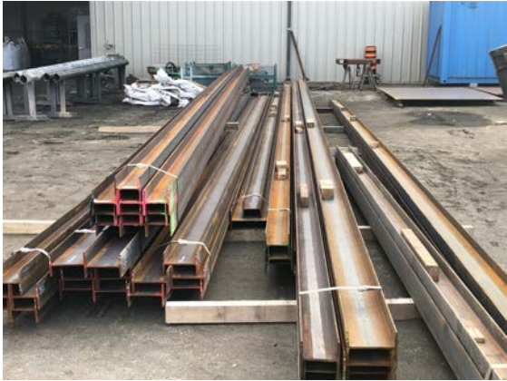
Steel delivery for piping modules
