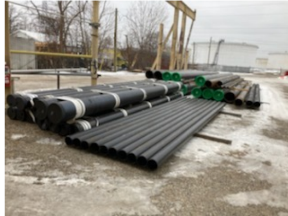
Piping delivery (approx. 12,000 linear feet of pipe)
