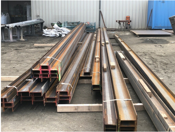
Steel delivery for piping modules
