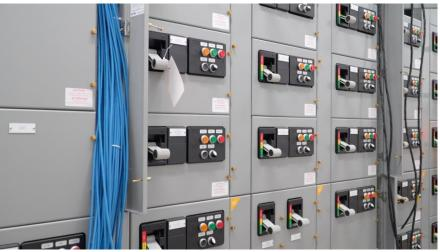
The power distribution building contains the motor control center
