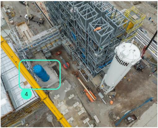
1. Storage tank for containing unrefined CMF before its distillation step. Due to its large size, our distillation feed tank was assembled onsite rather than delivered by road. The unpainted areas allow for welding. 2. Brine tanks and HCl tanks. 3. Solvent tanks and storage tanks for finished CMF. 4. Brine recovery tank
