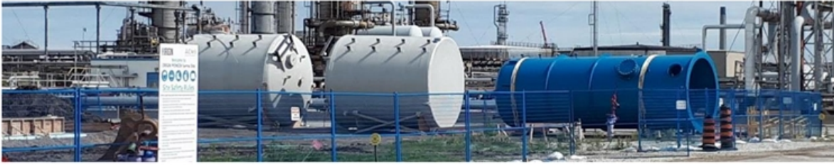
Tanks in construction yard
