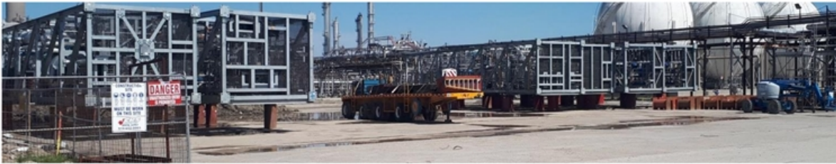
Core process modules awaiting installation
