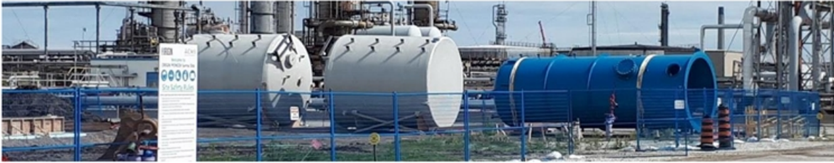
Tanks in construction yard
