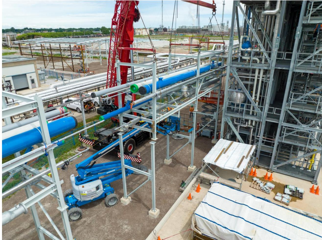
Piping modules have been interconnected alongside the plant's key production modules. They will move chemicals and materials through Origin's core chemical process
