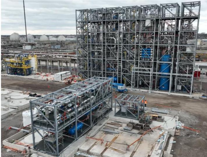
“After”: Clockwise from top we see the biomass building, HTC building and filter press, solvent tanks, piping modules
