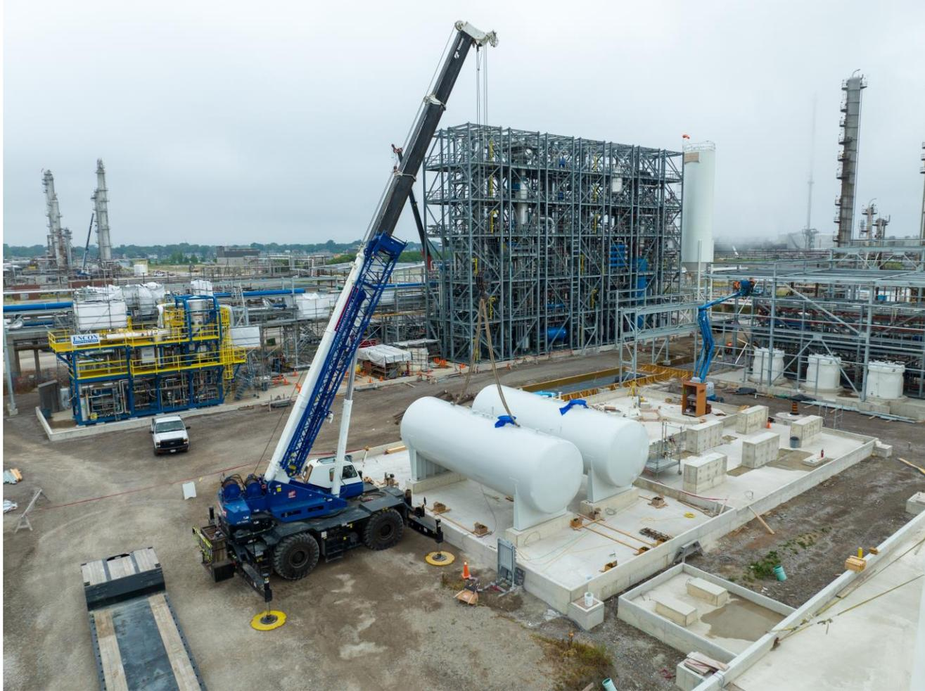
Storage tanks will contain solvent used and recycled in Origin's core chemical process
