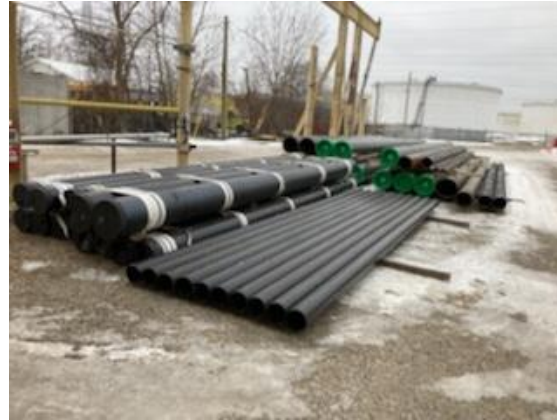
Piping delivery (approx. 12,000 linear feet of pipe)
