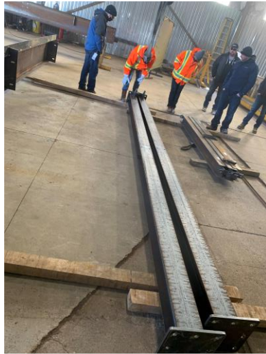
Finished steel verticals
