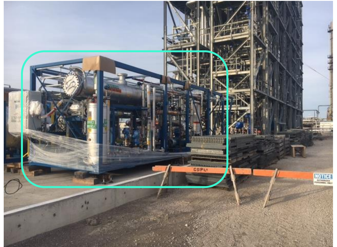
ENCON module system placed
