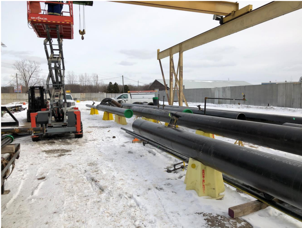
Pipe fabrication prior to painting
